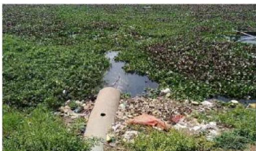
Fig. 2- Discharge from drains into Bara Talab, Bundu
